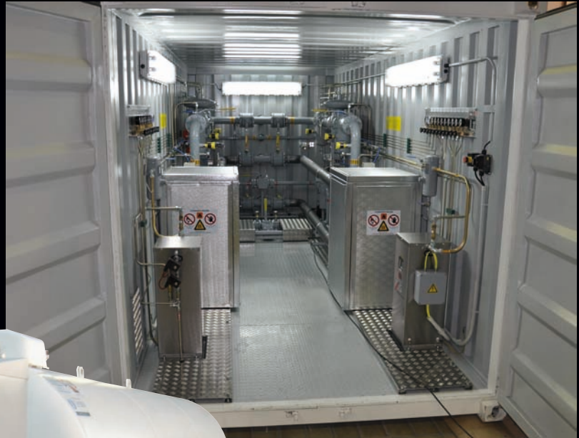
Examples of installations of vaporizer units
