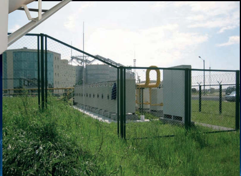
Examples of installations of vaporizer units
